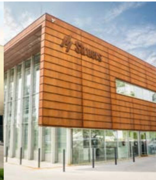
ROPER Engineering Built-to-Lease Lokalita Ostrava Plocha 4 400 m 2
